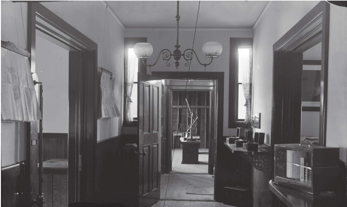
Gas chandelier in the hallway at Ladd. Early 1890s. (The line is a crack in the glass photographic plate.) Credit: Brown University Library / Archives.
