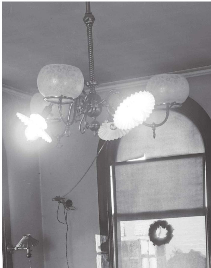
Closeup of the library chandelier. Note how crudely the wires were strung from the wall to the ceiling. The original gas lamps fixtures are partial globes. The electric lamps have fluted glass disks. Credit: Brown University Library / Archives.
